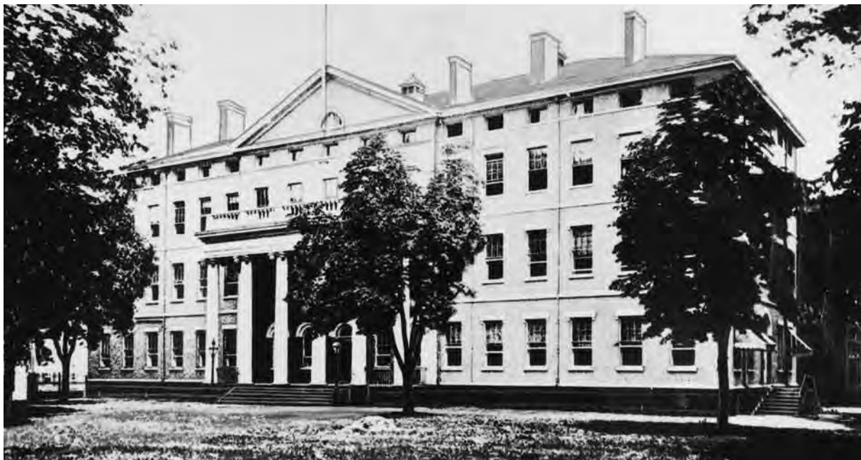
MODIFIED EXECUTIVE OFFICE BUILDING. At Secretary Stanton’s direction and with congressional approval and funding, two floors were added to Old War and Old Navy to meet Civil War expansion requirements. From Ingersoll’s History of the War Department (1880), reproduced by the Library of Congress.
